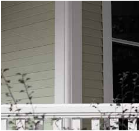
Trimworks® three-piece beaded corner post.
