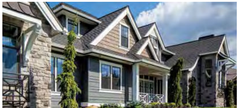
Featured: LP SmartSide Lap, Cedar Shakes (staggered), Soffit, Trim and Fascia
